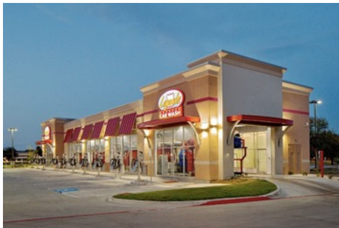
Express example (conveyor belt format) with self-serve vacuums
